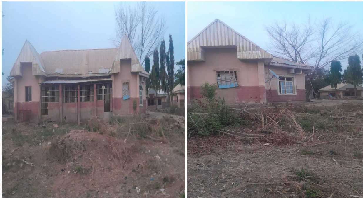
Figure 3: An example of setback violation to carnal (natural water lines) in Ikole. The implication to that violation is that this particular building is always submerging in flood every year
