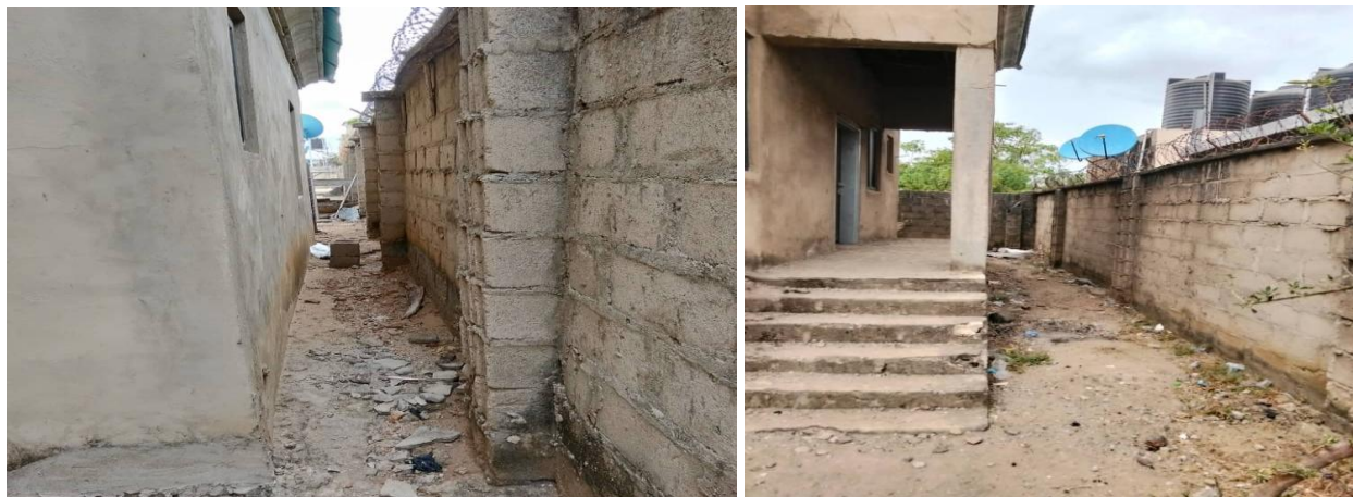
Figure 6: an example of building setback violation in Omuo. The setback to the side is 600mm and less than 2500mm to the front.
